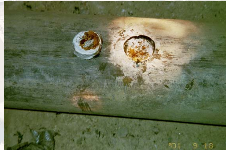
Hole in duct
