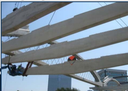
Hanging Floor Beams
