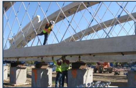
Hanger Tensioning
