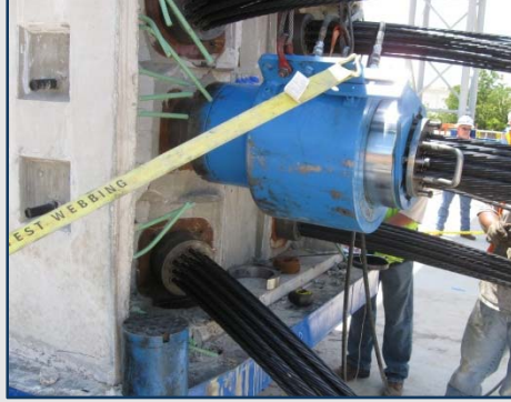
Hanger Tensioning
